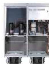
Fans under raised floor provide same air flow with 20% less power consumption
