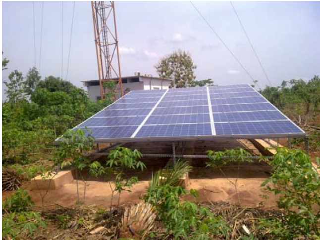
Figure 3. PV-hybrid PS installation in Togo
